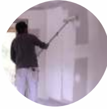
Birla Putty finished internal walls
